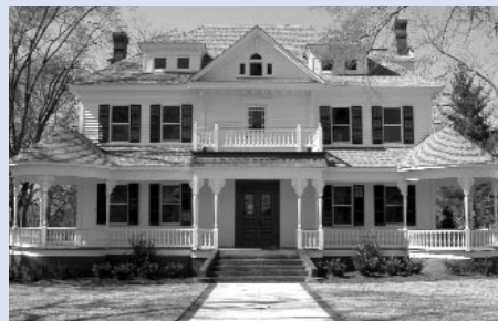
BRANTLEY-HAYGOOD HOUSE, Sander-ville, c. 1850/1890. This 5,400-sq.-ft. house has undergone a complete exterior rehabilitation: new roof, stabilized foundation, extensive wood repair, new paint, rebuilt chimneys and landscaping. Interior work has not been completed. Features hardwood floors, Victorian-era mantels and original doors. Sits on a 1-acre lot. Listed on National Register. $245,500. Contact Frank White at 404-885-7807.
